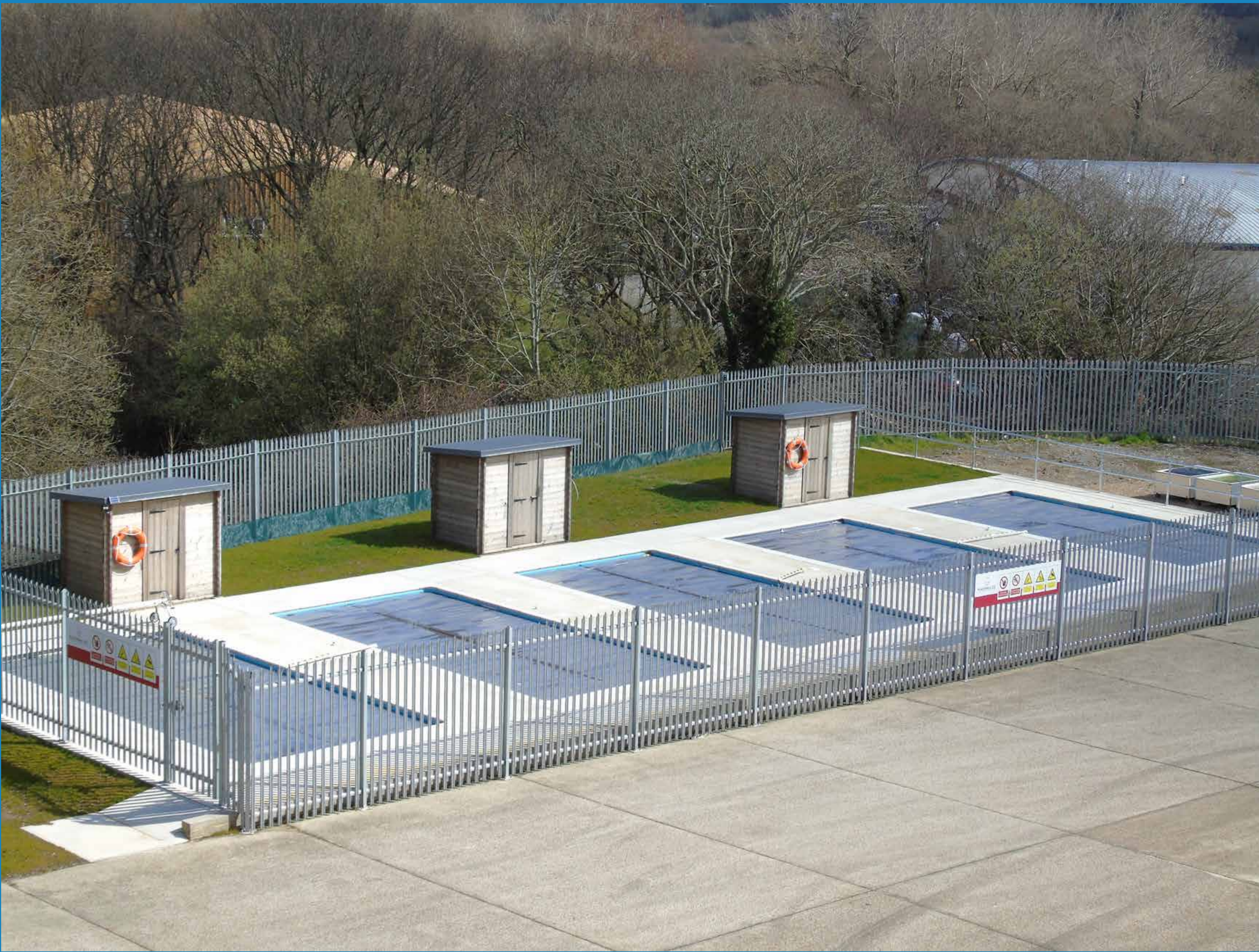
Figure 3. Bespoke testing facility, Plastipack Ltd, Hastings UK.
